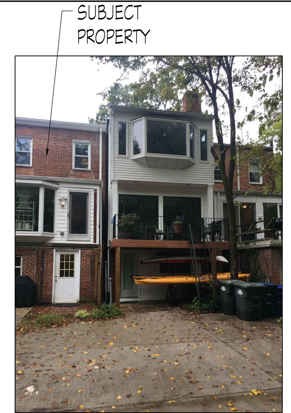
4 VIEW OF REAR LOOKING WEST TO PROPERTY TO THE NORTH, LOT 78
