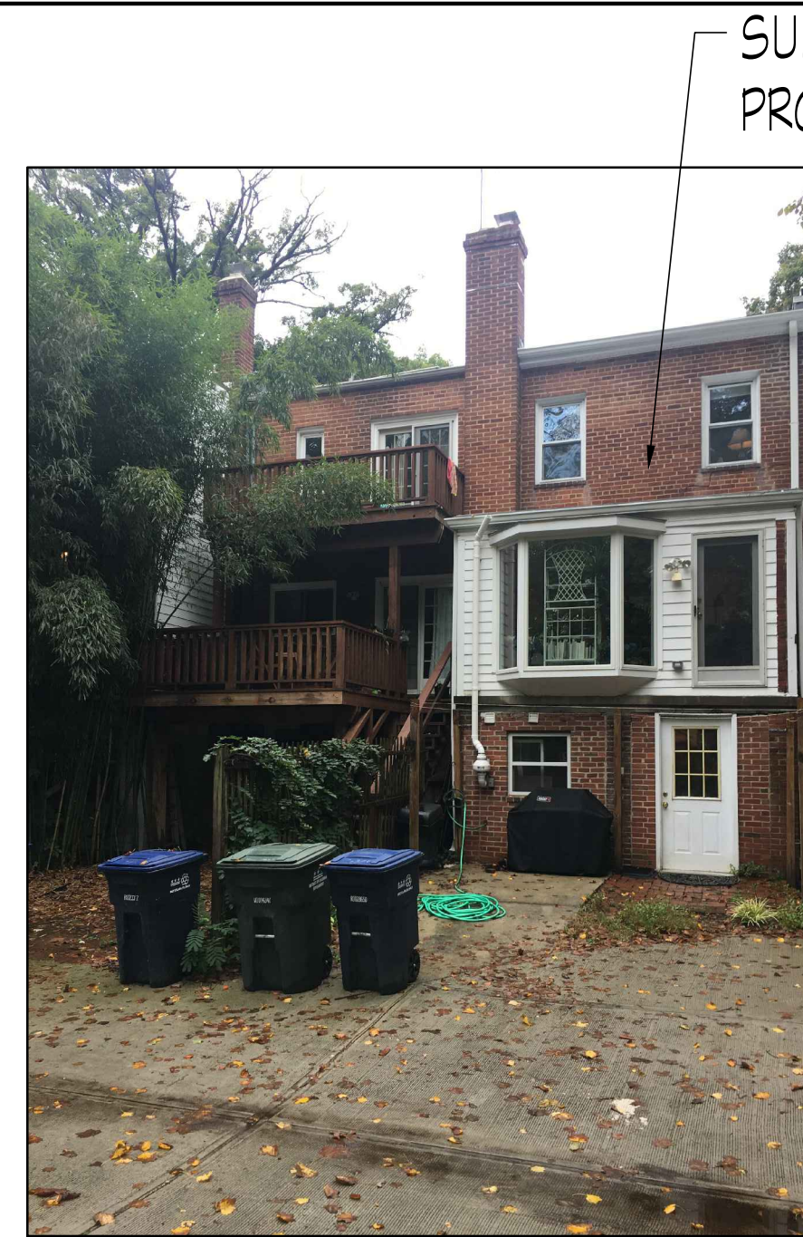
2 VIEW OF REAR LOOKING WEST TO PROPERTY TO THE SOUTH, LOT 76
