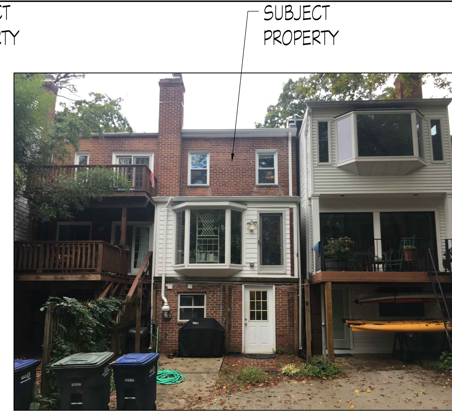
3 VIEW OF REAR OF PROPERTY LOOKING WEST
